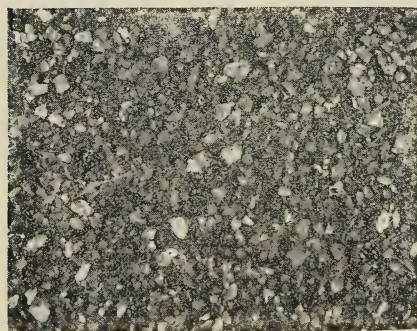
FIG. 126.—Prepared Roofing Finished with Crushed Feldspar.
